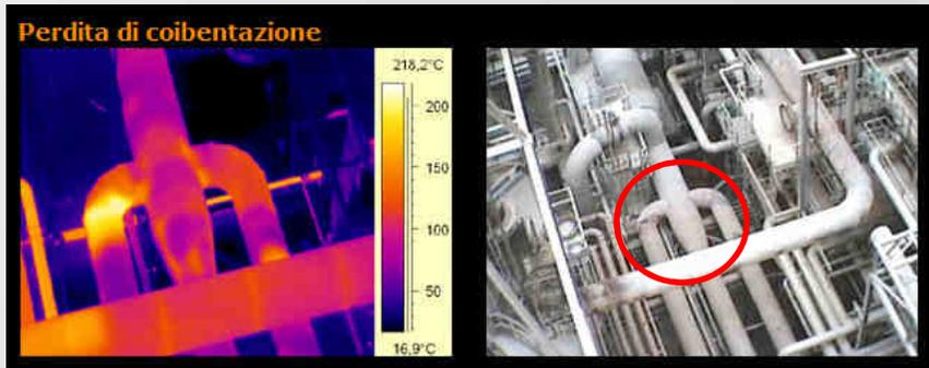
**PIPING SYSTEM: LOSS OF INSULATION ON PIPING (1)**
