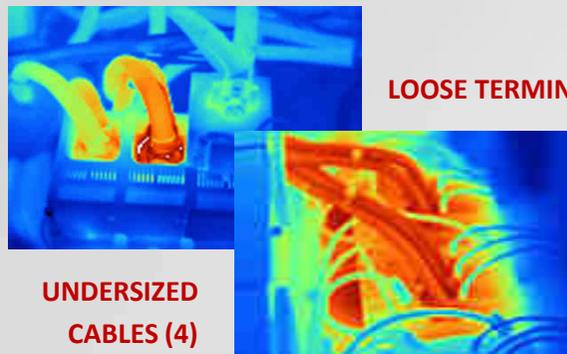
These pictures show others thermographic measurements but, in this case, we can see industrial equipment. Especially in the existing plant systems we can find conditions such as those represented in the images. Inefficiencies due to damaged insulation or insulation evil placed, incorrectly connected terminals or undersized cables.
